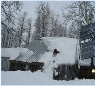
Snow avalanching off Yentna Station roof.
